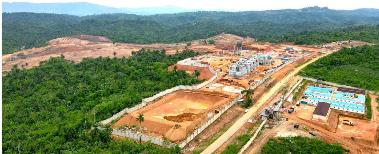
Segilola Project Construction Overview (June 2021, Thor corporate presentation )
